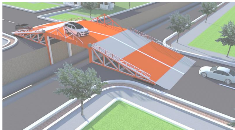
Fig. 2. - Modular communal overpass
