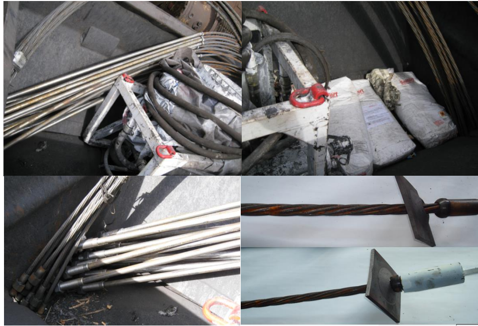
Fig. 6. – Roof bolting of the JV Minova-Kazakhstan LLP (rope anchors)
