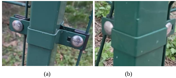
Fig. 2. Metal clamps available on the market; (a) clamp for indirect (parallel) connections, (b) clamp for angular (perpendicular) connections
