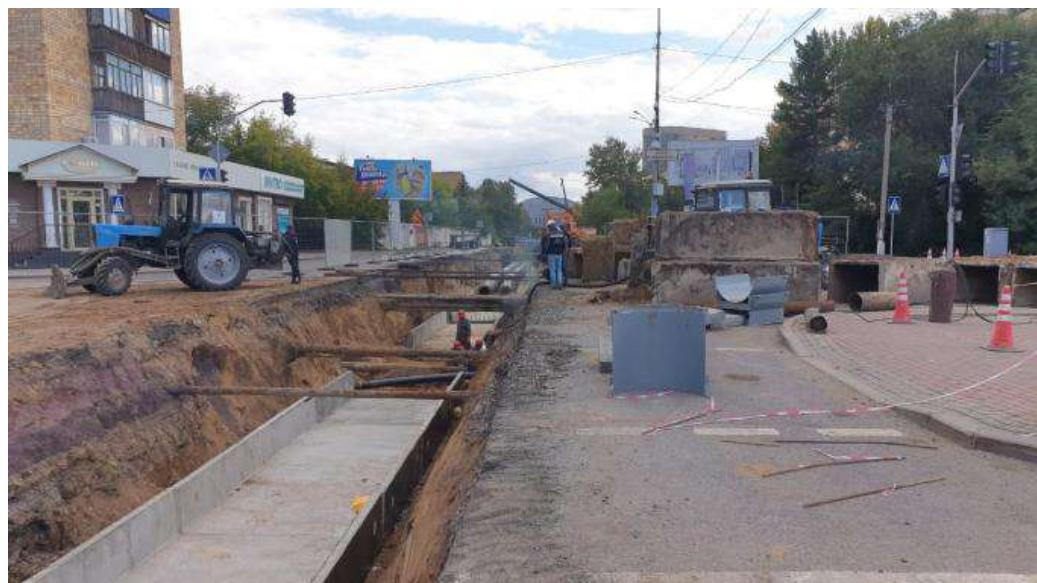
Fig. 7 – Work on replacing utilities (pipelines)
