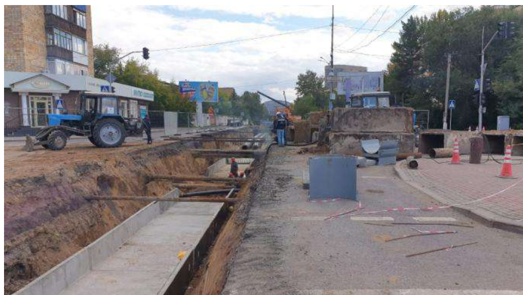
Fig. 7 – Work on replacing utilities (pipelines)
